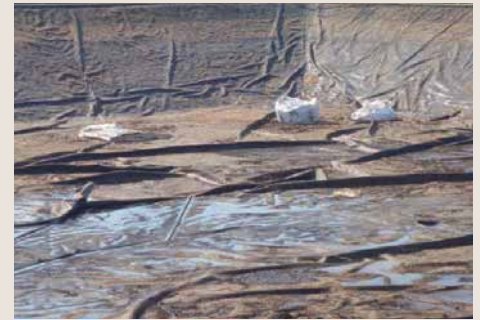
Pond empty for HDPE liner repair
