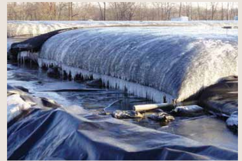
Dewatering under winter conditions
