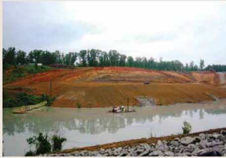
Reclaimed site after dewatering
