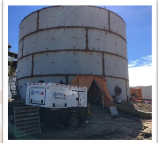
Delivering hot, dry, air to control humidity and temperature while coating a large tank
