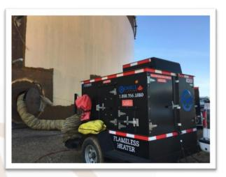
A single CH15HS heat<mark>er pro</mark>viding hot, dry air to cure coating on a large tank eve<mark>nly w</mark>hile keeping workers warm
