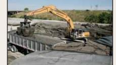
Dewatered sludge being removed from a Geotube® container with an excavator
