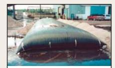
Coal sludge dewatering using Geotube® dewatering technology
