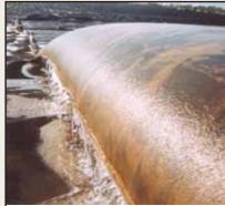
Water draining from a Geotube® container.
